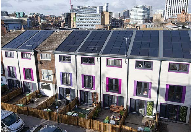
ENERGIESPRONG NET ZERO RETROFIT IN NOTTINGHAM, UK, 2019 - ENERGIESPRONG INTERNATIONAL, VIA FLICKR
