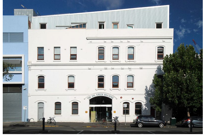
THE AUSTRALIAN CONSERVATION FOUNDATION'S 60L GREEN BUILDING, CARLTON, MELBOURNE - ELEKHH
