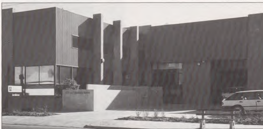
The new Archives climate controlled repository, Dawson Street.
