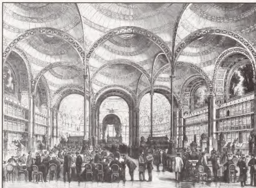
The Reading Room of the National Library, Paris, illustration by Henri Labrousse: the roof "cupolas" are of enamelled porcelain and the room was heated via hot-air pipes at the feet of the readers. It housed 40,000 volumes (from the Illustrated London News , collection of the author).
